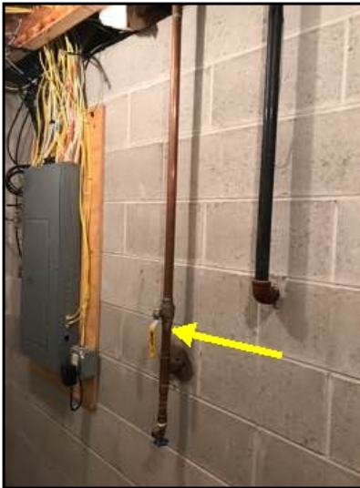
Water shut off for irrigation system.
