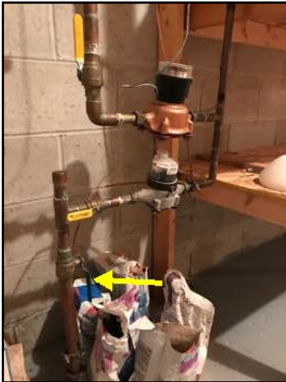
Main water supply shut off.
