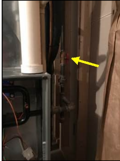
Gas shut off valve.
