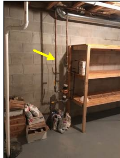
2nd line feeds irrigation system.
