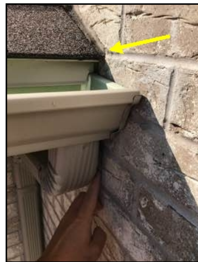
Brick spalling due to missing kick out flashing above garage door.
