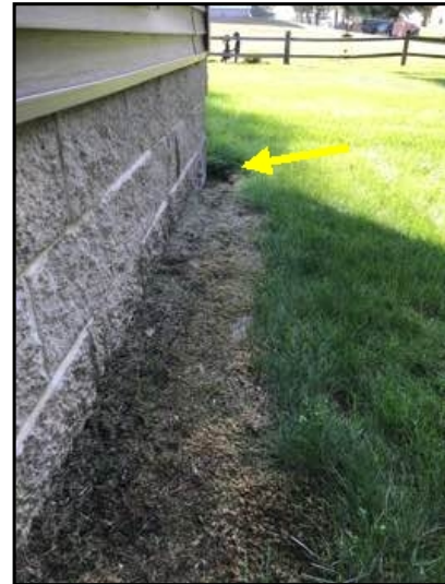
Small depression. NW. Back fill recommended.
