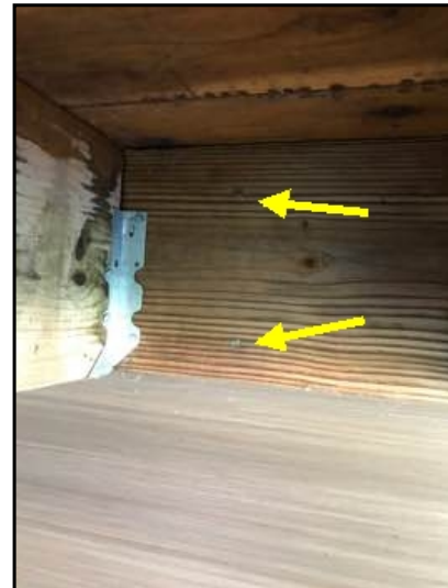
Ledger board anchored to house with deck screws. Lag screws are recommended.
