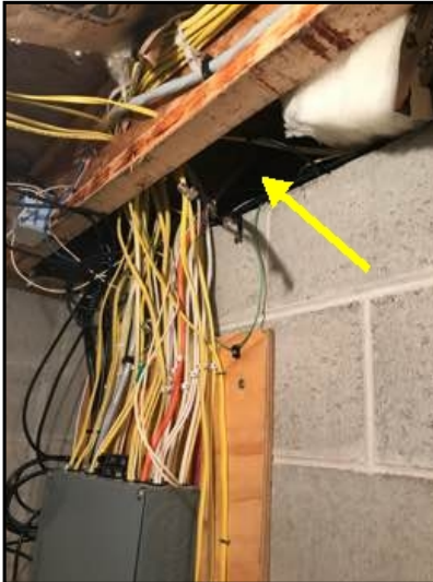
Missing insulation above electrical panel.
