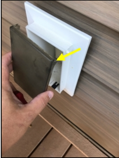
Deck outlet cover is damaged.
