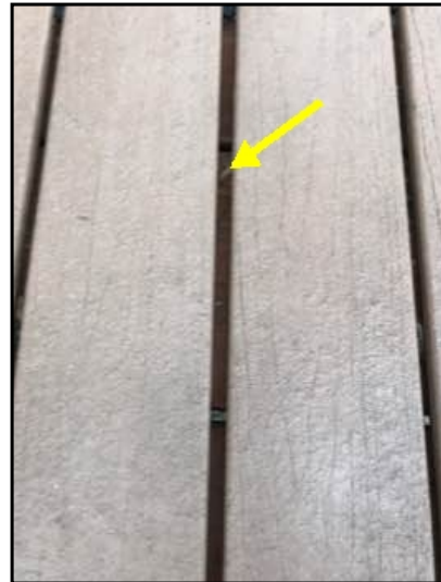
Composite decking installed over finished wood decking.
