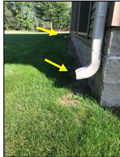
Downspout extensions recommended. North.
