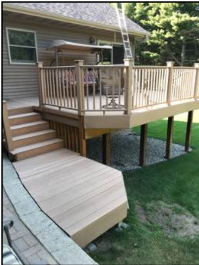
Wood to ground contact. footings were not visible or accessible.
