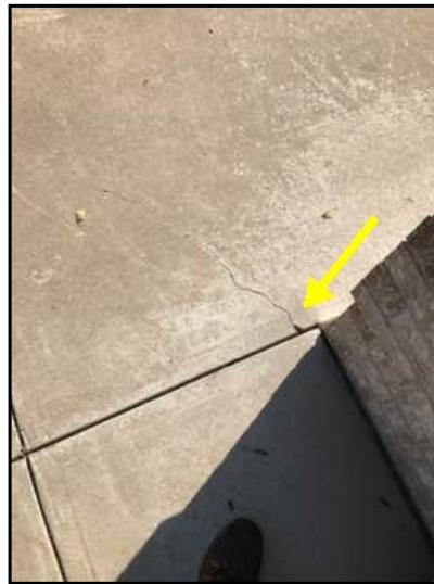
Small settlement crack at single garage door entry.
