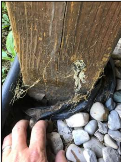
Wood to ground contact. footings were not visible or accessible.
