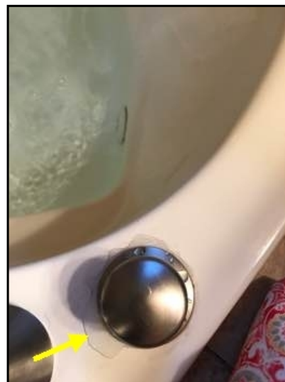
Shower head control has a small leak when depressed for shower head.
