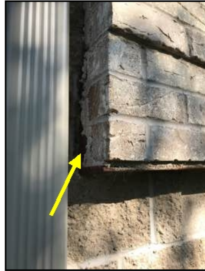
Gap in mortar. SW corner.
