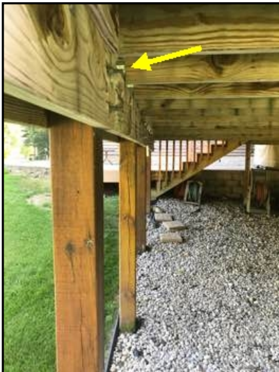
Lag bolted through vertical supports.
