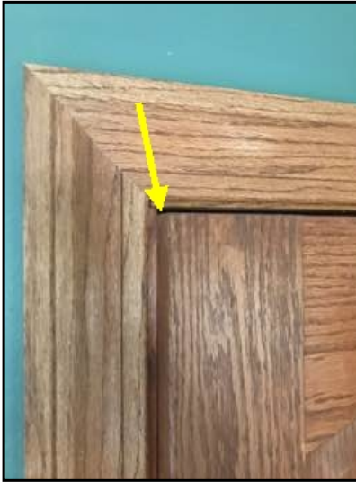
Door binding in frame at top corner.
