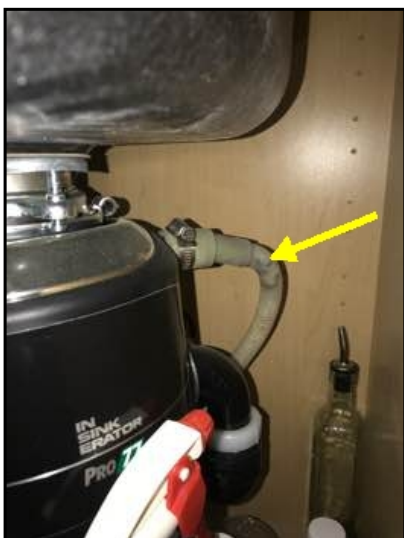
No high loop on dishwasher drain.
